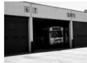
Sample Transit Facility.
